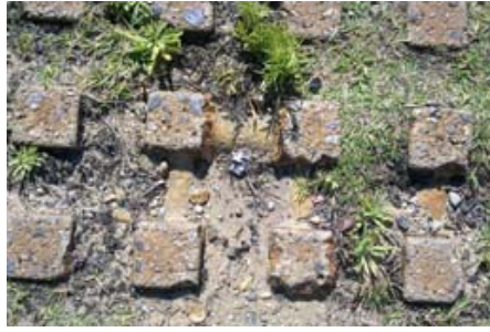
Figure 2: Concrete Grid Pavers near Canning Bridge, Western Australia
