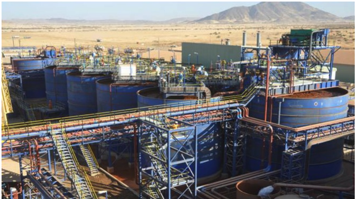
Figure 1.1. CIL tanks in series in a gold extraction plant in Eritrea, Africa (Resources, 2010).
