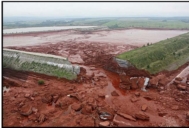
Figure 2.2 Hungary Tailings dam failure
