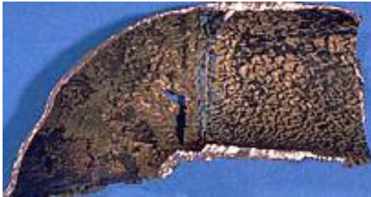
Figure 2.15: “Horseshoe” erosion-corrosion damage in a copper pipeline (Obanijesu et al, 2011d)
