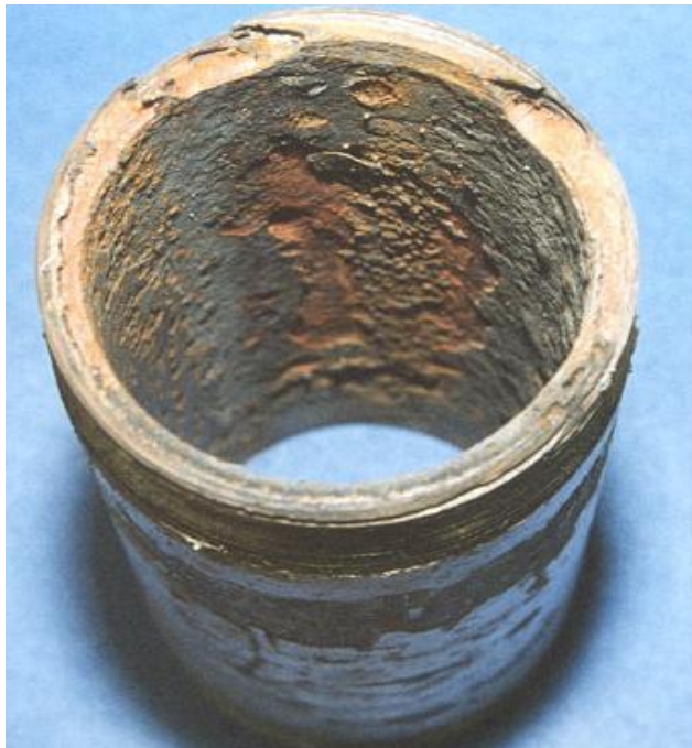
Figure 2.18: A metal attacked by crevice corrosions (Obanijesu et al, 2010c)
