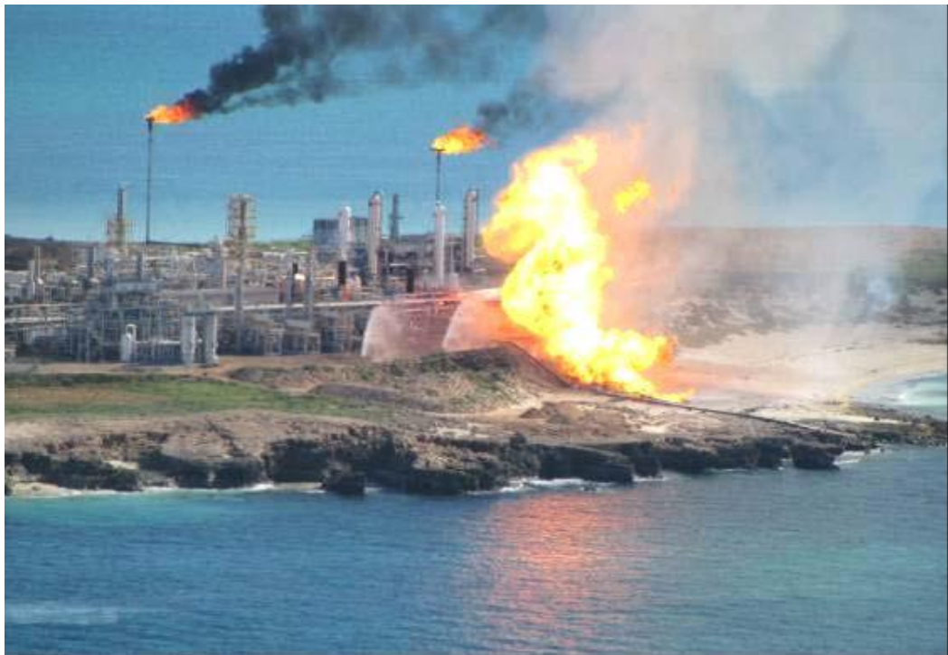
Figure 2.23: Veranus Island pipeline explosion (Cutler, 2010)
