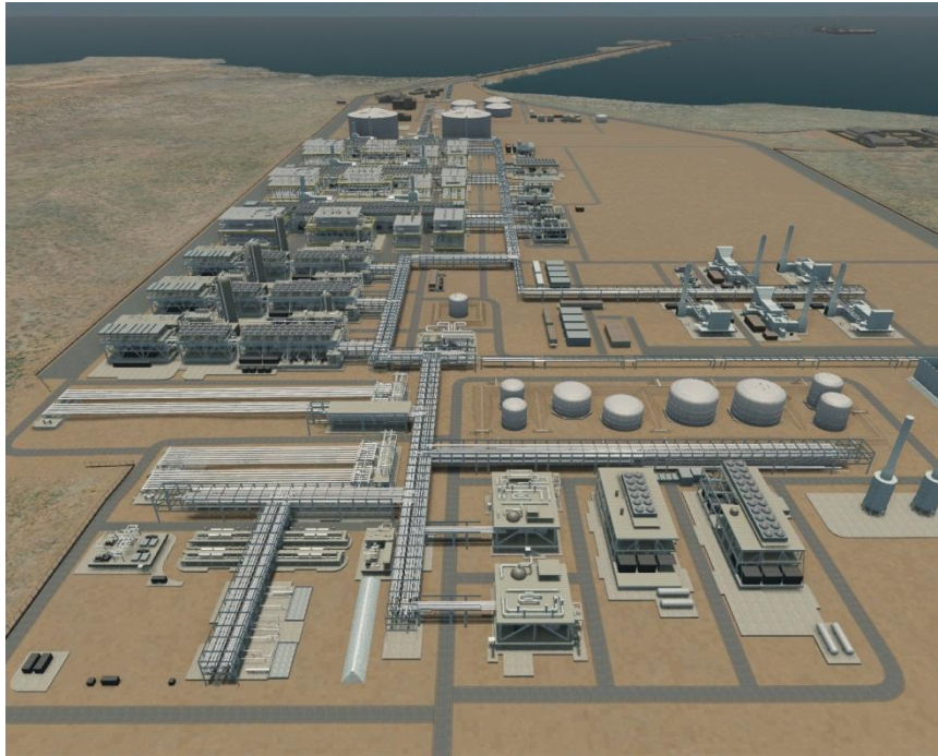
Figure 2.8: The gas treatment facility at Barrow Island
