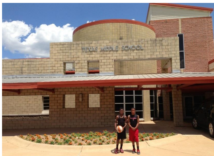
Figure 3.1: Texas Middle School, Texarkana, Texas
