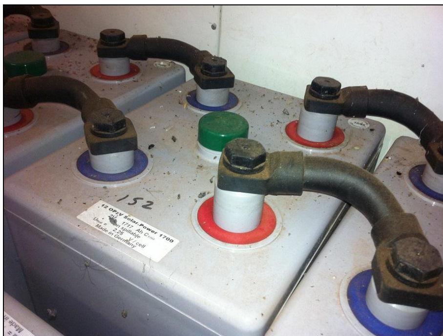
Figure 5. 8: Damaged Battery
