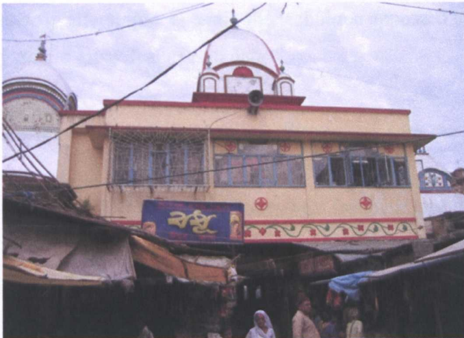
Fig. 6.13 Kalighat mandir administration offices above the main entrance to the mandir
