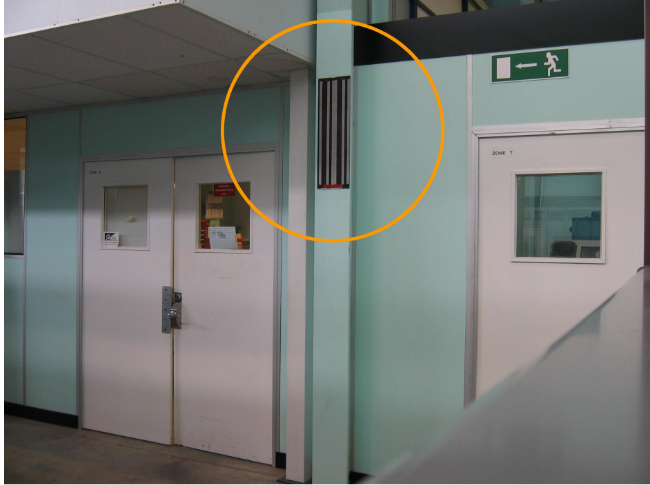
Figure 2.5: Artificial landmark for a factory Autonomous Guided Vehicle (AGV), comprised of a barcode of retroreflective strips.
