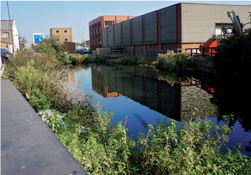
Shackles Dock canal inlet
