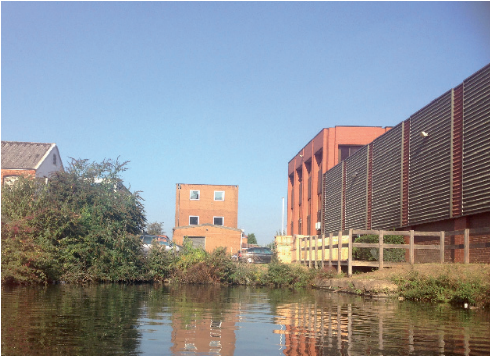
View into Shackles Dock from the canal inlet
