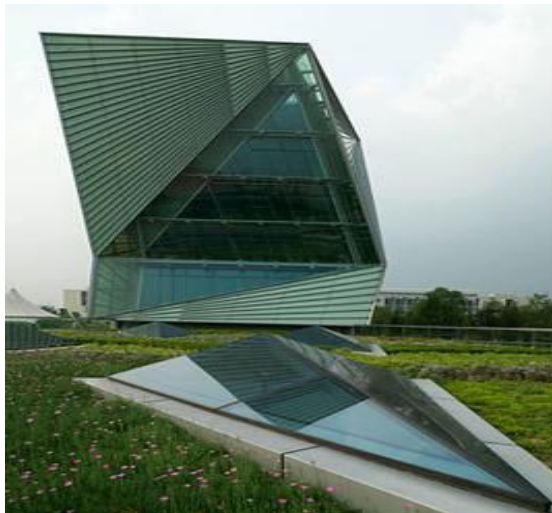
Figure 1. A view of the green roof on top of the lab spaces in the CSET building in Ningbo
