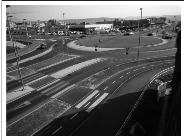
Figure 1 - Turbo roundabout; City of Koper, Slovenia
