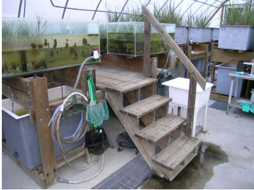
Figure 26: Stairs added to end of platform
