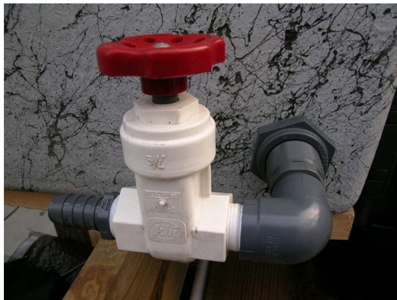
Figure 6: Tidal Exchange plumbing (exterior) completed
