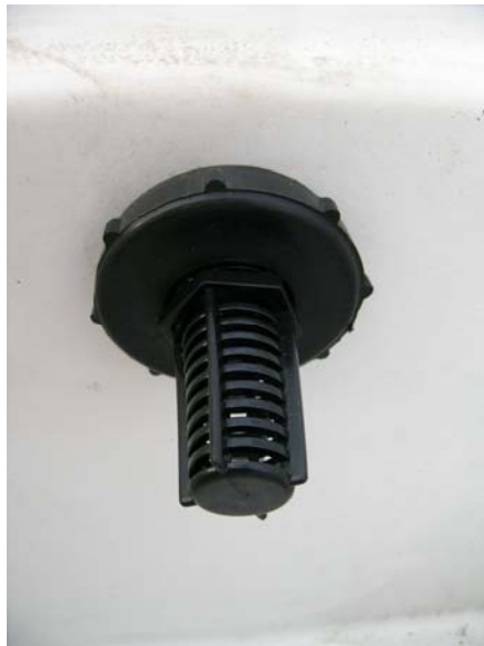
Figure 11: Overflow plumbing (interior)
