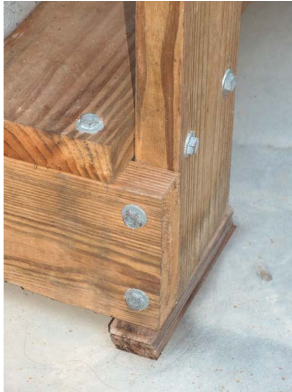
Figure 25: Picture showing the 3-dimensional pin attachment
