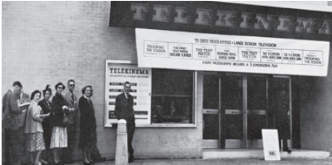
ABB. 1.19 Außenansicht Telekinema, London, South Bank Exhibition 1951
