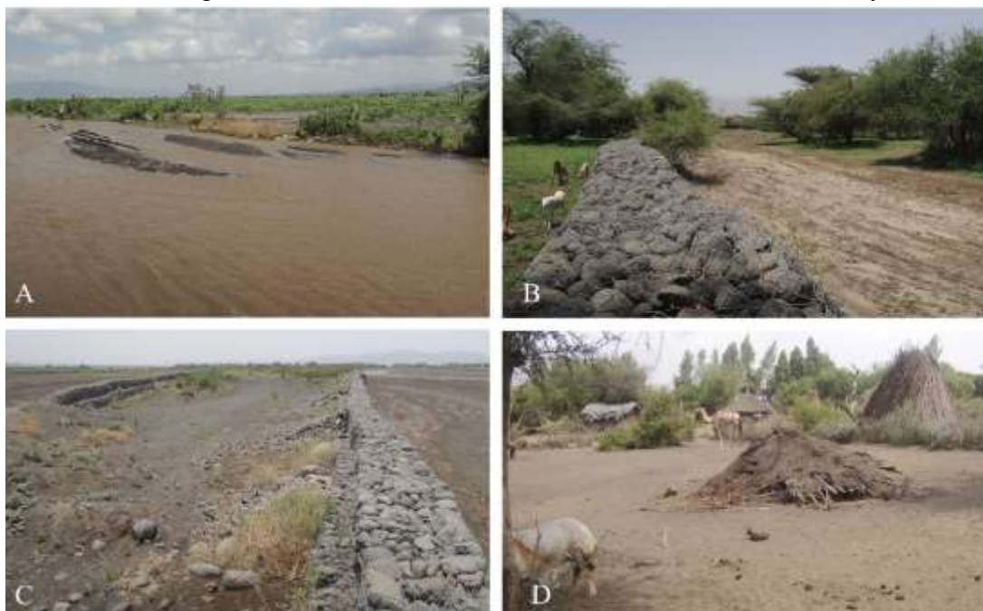
Figure 5. Land management practices in the graben bottom related to rivers: (A) traditional land management practices; (B) gabion structures for protection from flooding; (C) gabion dykes to protect Waja town; and (D) the Gubena village, covered with metres-thick sediment of Gobu River. Note the roof of a house emerging above the sediment; the people moved to the new house behind it.
