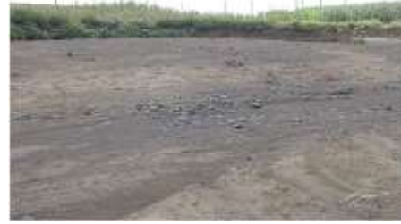
Figure 3. Bank erosion in upstream reach of Oda River. The flow direction is to the right of the photo.
