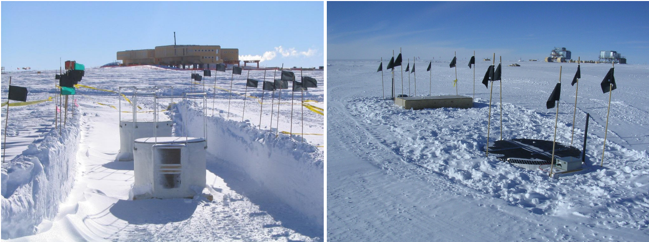
Figure 2.10: An IceTop station during deployment in an open trench (left) and when the trench was refilled with snow (right).
