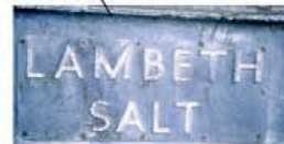
Eroding: Street Cleaning Road Salt Dispenser
