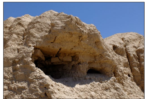
Figure 5: Cavities at the top of the southwest corner, which could correspond to the position of beams supporting a turret (Photograph Sébastien Moriset).
