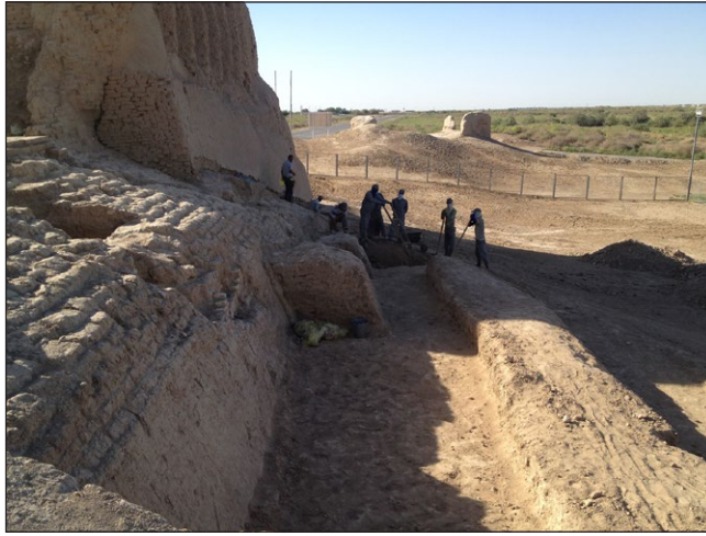
Figure 14: Eastern side of the Great Kyz Kala looking north, during excavation by the Park. Note the fair face to the skirt/glacis (to the left), and the buttresses constructed along the northern part of the façade (centre). The decreasing height of the buttress/pillars to the north reflects erosion patterns, rather than necessarily reflecting their original size. To the right the long wall parallel with the façade is just beginning to be cleaned (Photograph Paul Wordsworth).
