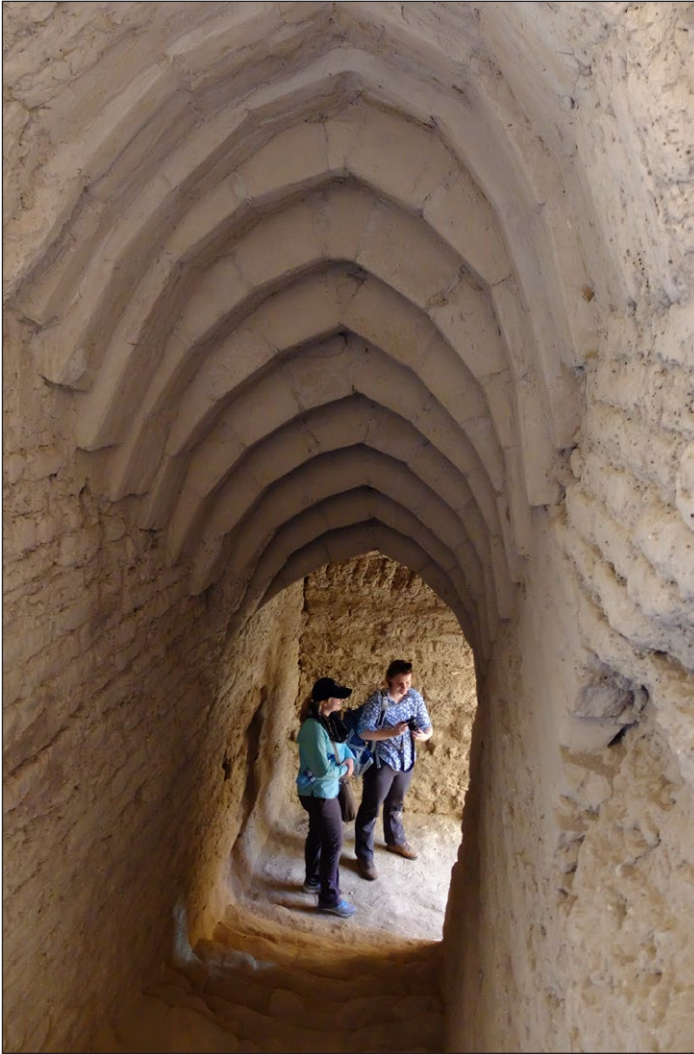
Figure 13: Internal staircase, roofed by a series of stepped tunnel vaults, leading down from second storey to the courtyard (Photograph Sébastien Moriset).
