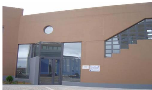
Figure 1 The Maintenance Support building of Technical University of Crete
