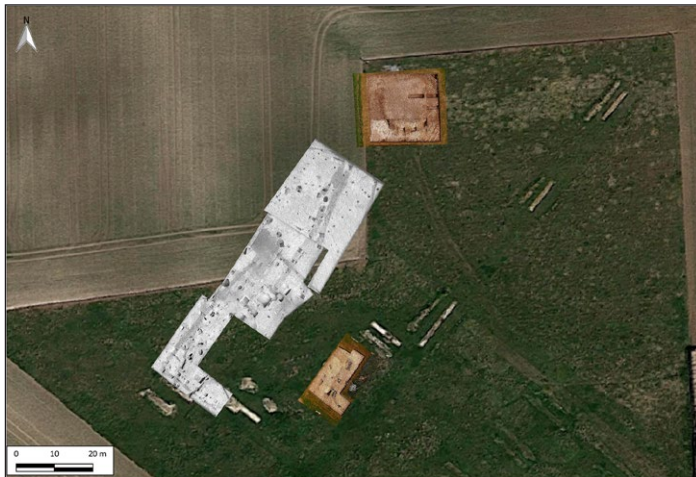
Figure 4: Aerial image, showing the position of the existing excavations 2015–18. [Base layer Google Earth. Rob Kaleta/Downley Project].
