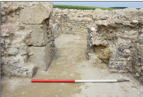
Figure 6: Detail of the construction showing dressed Caen stone, Upper Greensand wall-fill, and dressed flint internal facings. (Scale 0.5 m divisions). Photo: MBR.
