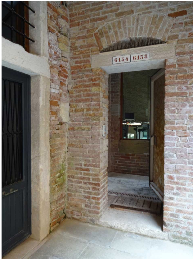
Figure 8.1 The door which enticed us
