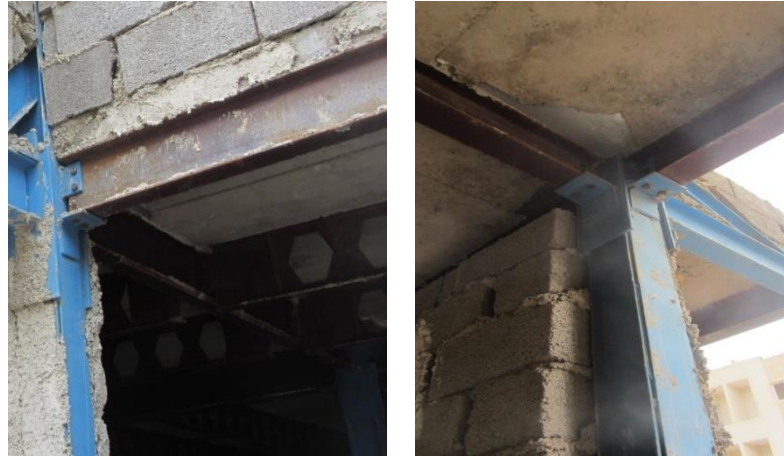
Figure 5.20 - Beam-column connection of the index building
