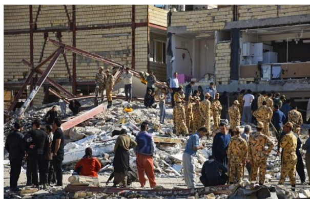
Figure 1.5 – Collapsed steel building in Sar-pole-zahab, observed during 2017 Iran-Iraq earthquake
