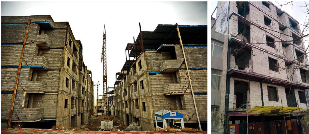
Figure 1.1 - Samples of masonry infilled steel frame projects under construction in Iran
