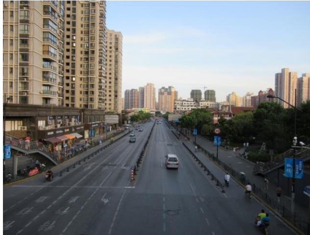
Figure 12: Example of community severance caused by a large urban road
