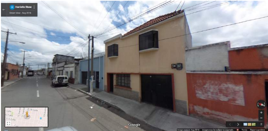
Figure P-50 Building 9: Omni-directional image – view 1
