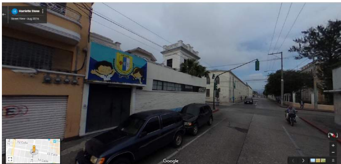
Figure P-15 Building 3: Omnidirectional image, view 2
