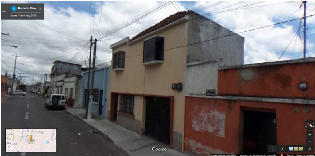
Figure P-52 Building 9: Omni-directional image – view 3
