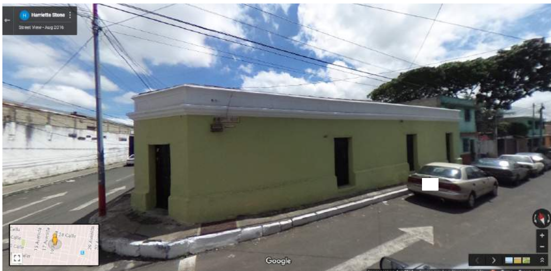
Figure P-44 Building 8: Omnidirectional image – view 2
