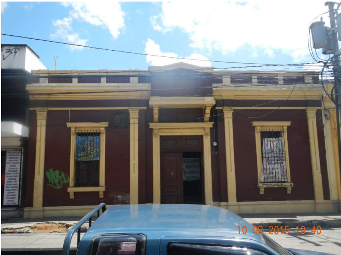
Figure L-1 Building 1: Street level photo of Colegio Mixto Santa Sofia
