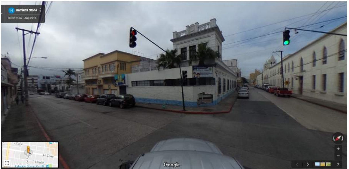
Figure P-14 Building 3: Omni-directional image, view 1
