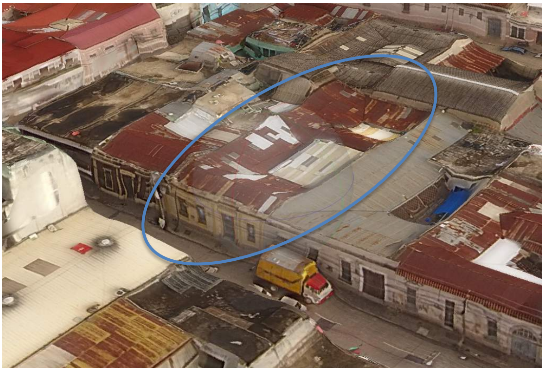
Figure P-36 Building 6: 3D model - view of building 6 from the south east
