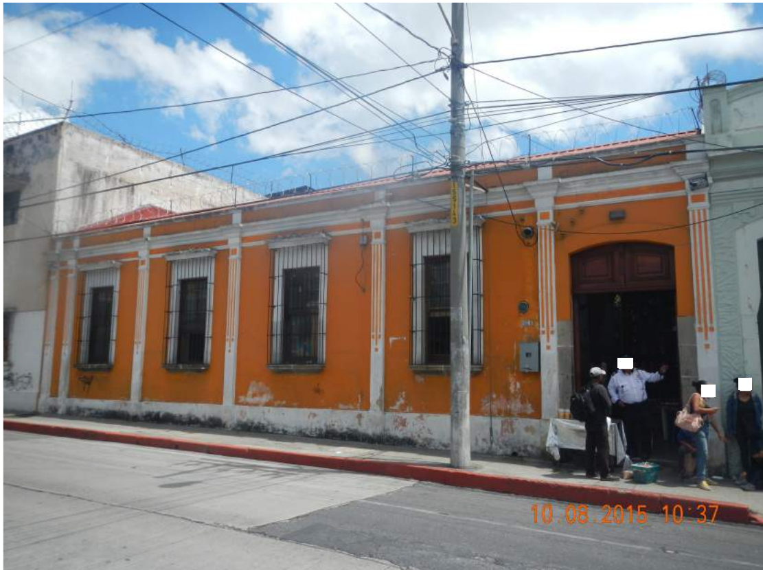
Figure P-27 Building 5: Street level view of building 5
