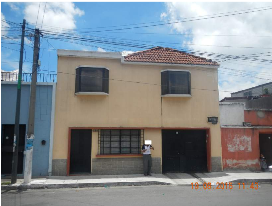
Figure P-49 Building 9: Street level view of building 9
