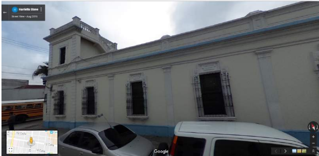
Figure P-16 Building 3: Omni-directional image, view 3
