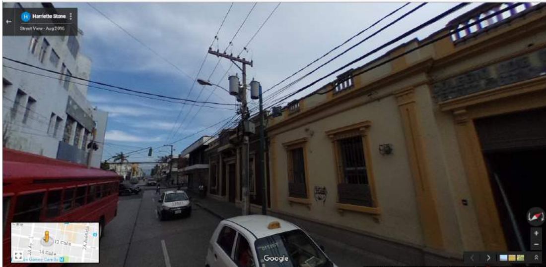
Figure L-2 Building 1: Omni-directional image - view 1
