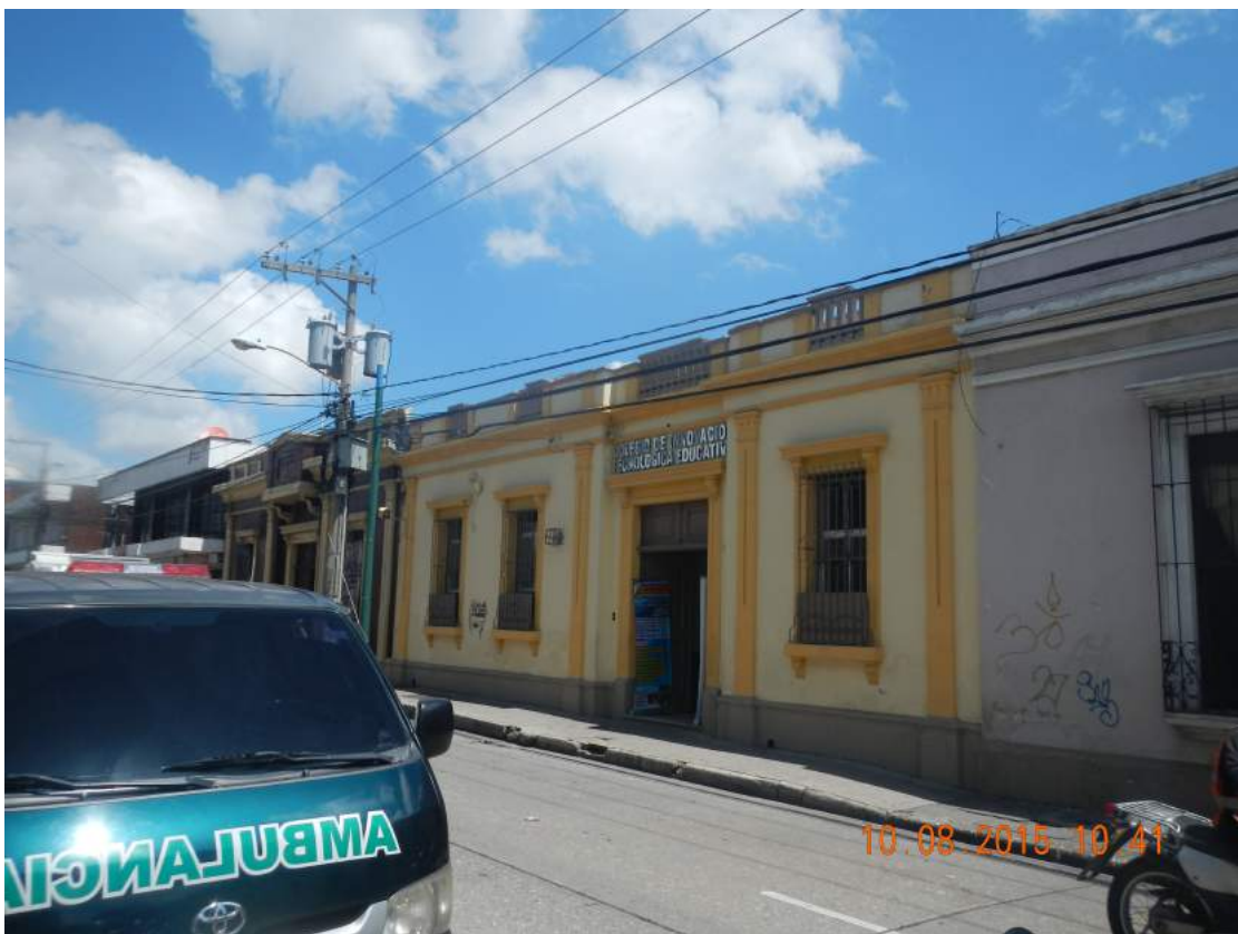
Figure P-32 Building 6: Street level view of building 6
