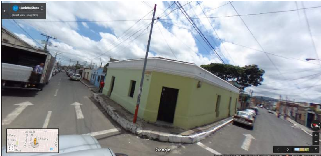
Figure P-43 Building 8: Omnidirectional image – view 1
