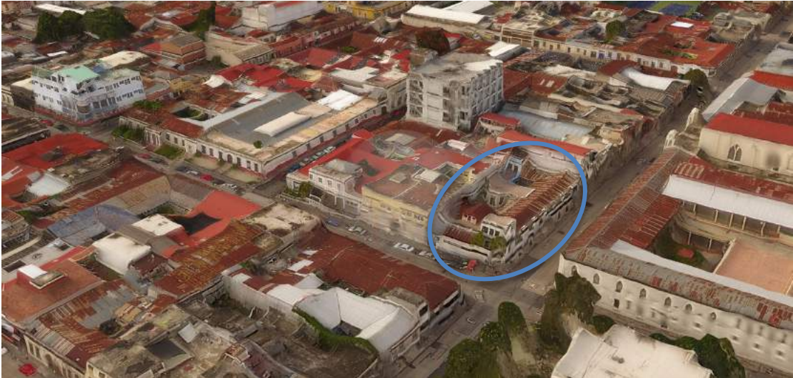
Figure P-18 Building 3: Drone 3D model – building 3 from the north west
