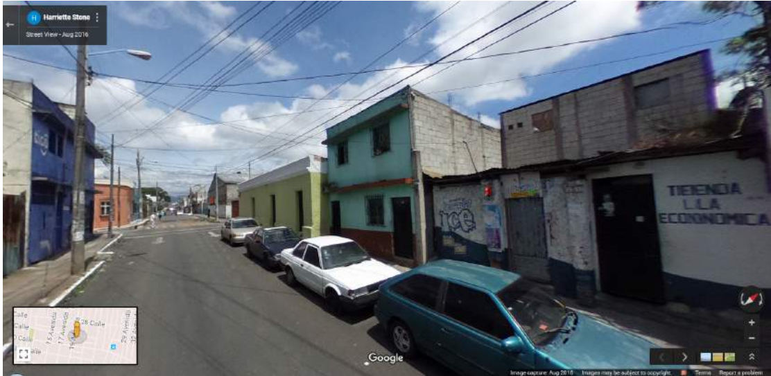
Figure P-45 Building 8: Omnidirectional image – view 3
