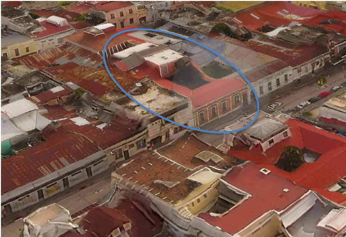
Figure P-29 Building 5: 3D model – view of building 5 from the south west
