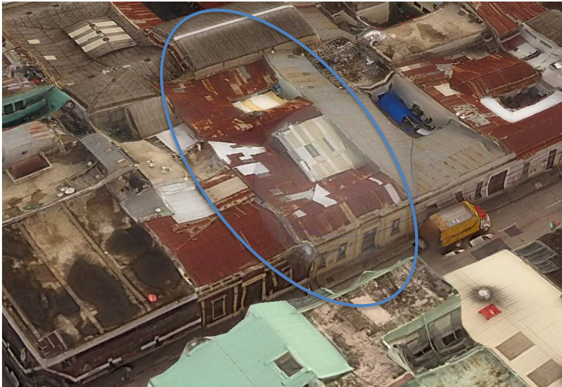
Figure P-35 Building 6: 3D model – view of building 6 from the south west
