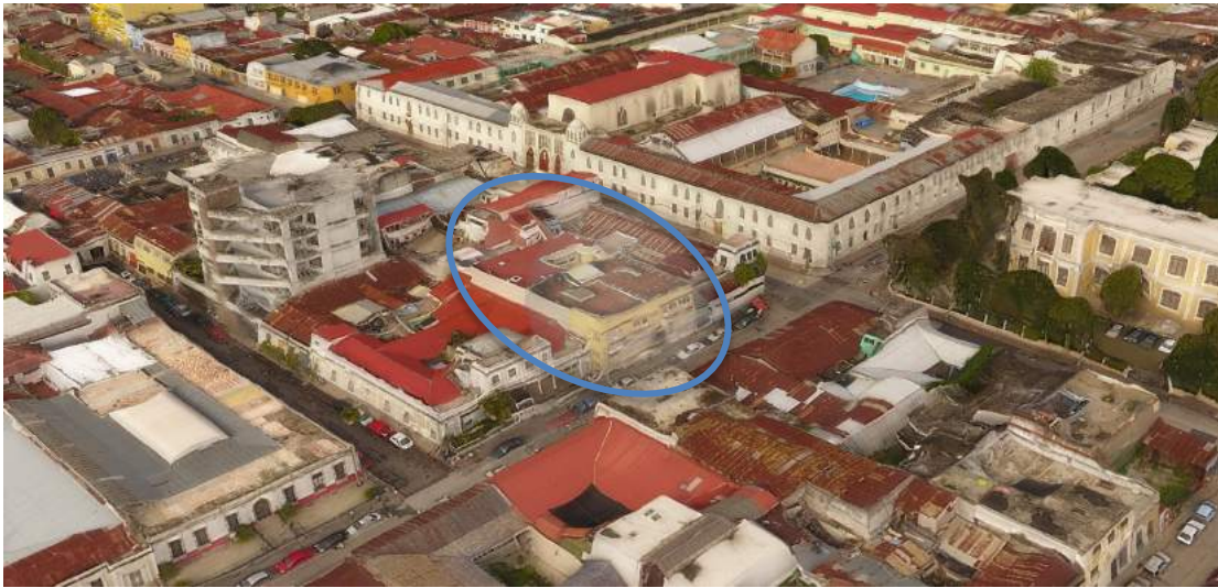
Figure P-10 Building 2: Drone 3D model - Instituto de estudios comparado ciencias penales de Guatemala from the north east
