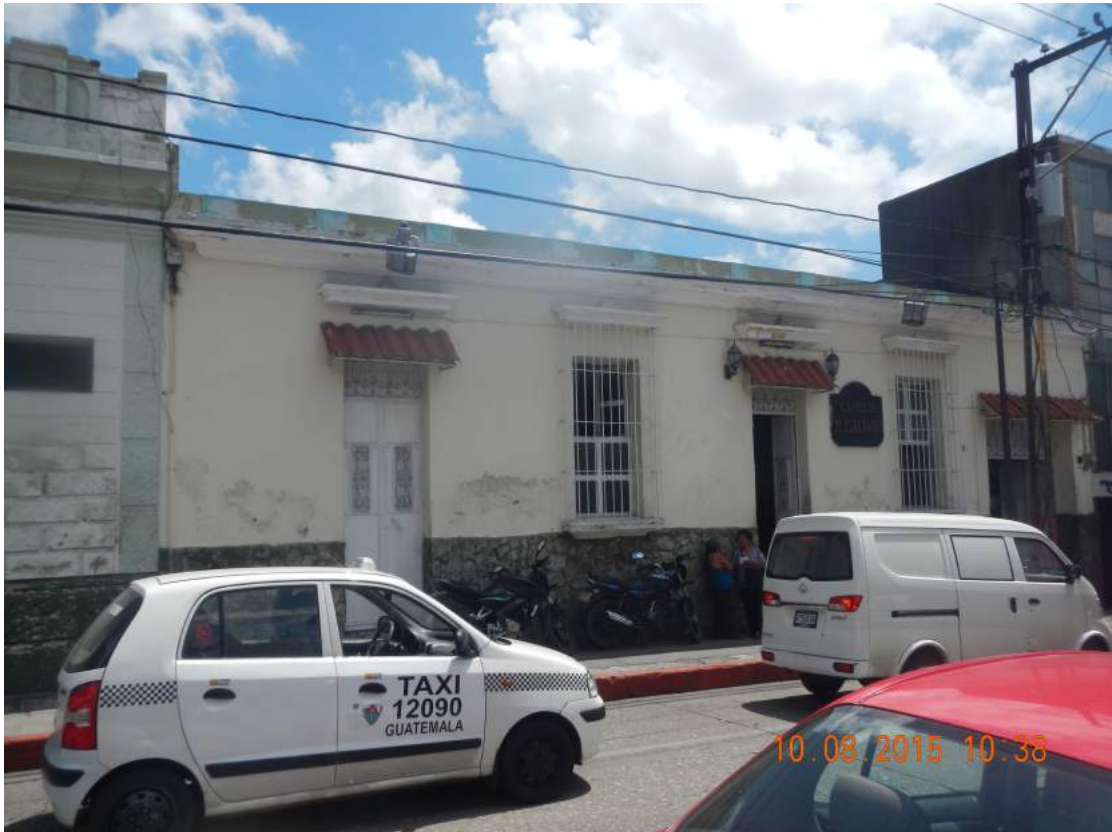
Figure P-21 Building 4: Street level view of building 4
