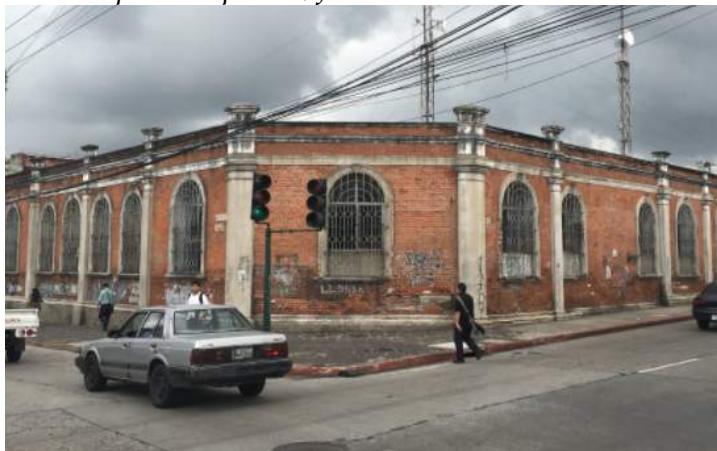
Figure 5-27 The electrical company building in September 2016. The building was reduced to a single storey structure after the earthquake.
