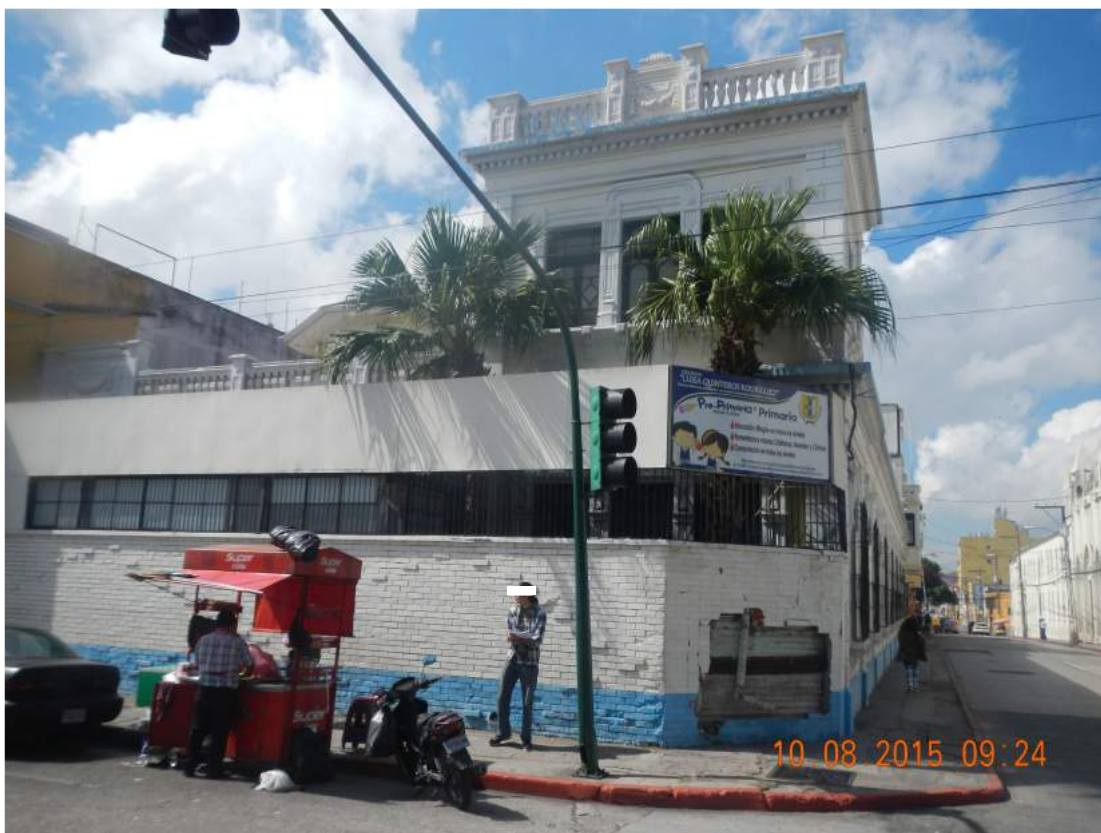
Figure P-13 Building 3: Street level view of building 3
