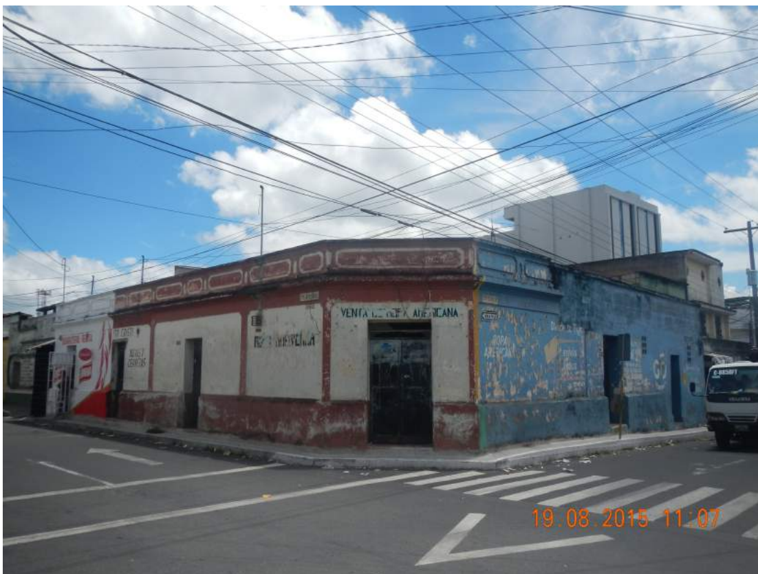
Figure P-37 Building 7: Street level view of building 7
