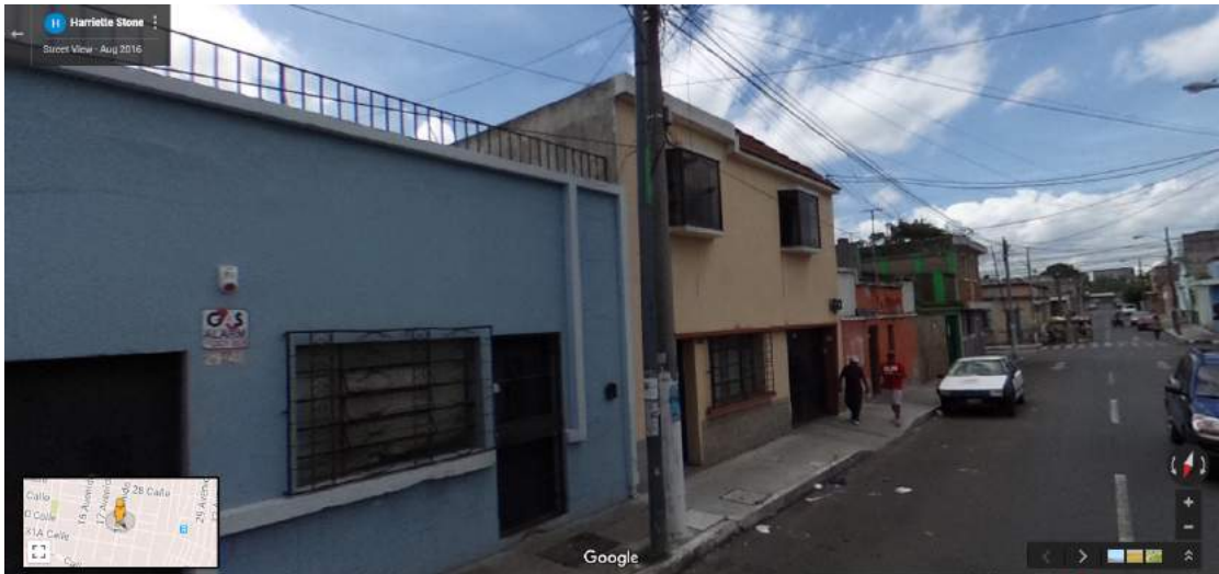
Figure P-51 Building 9: Omni-directional image – view 2
