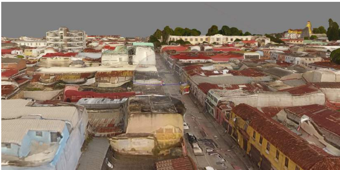
Figure 5-6 Looking west along Calle 13, Zone 1, Guatemala City: an example of a 3D tiled point cloud model constructed from UAV imagery
