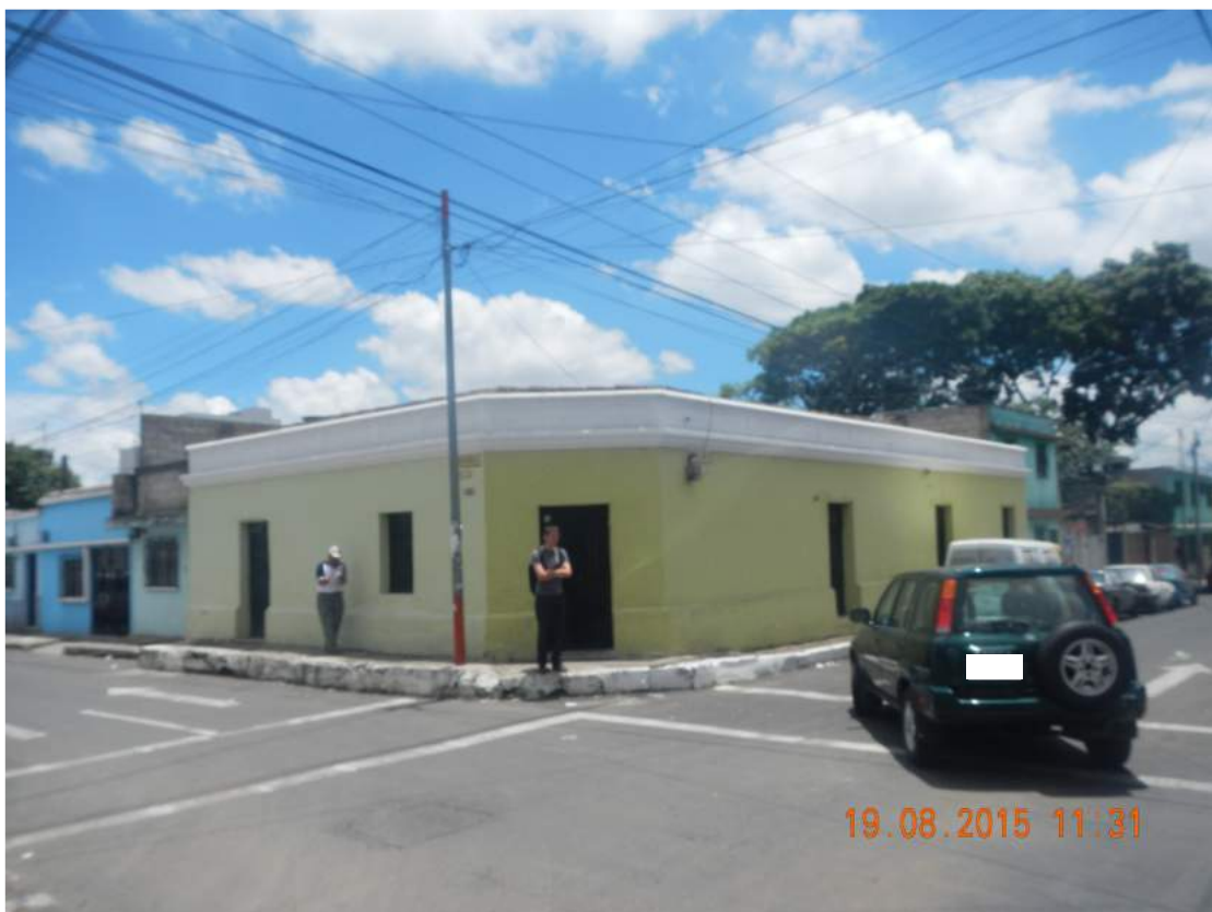
Figure P-42 Building 8: Street level view of building 8
