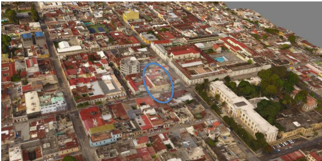
Figure L-9 Building 2: Drone 3D model - The neighbourhood around the Instituto de estudios comparado ciencias penales de Guatemala
