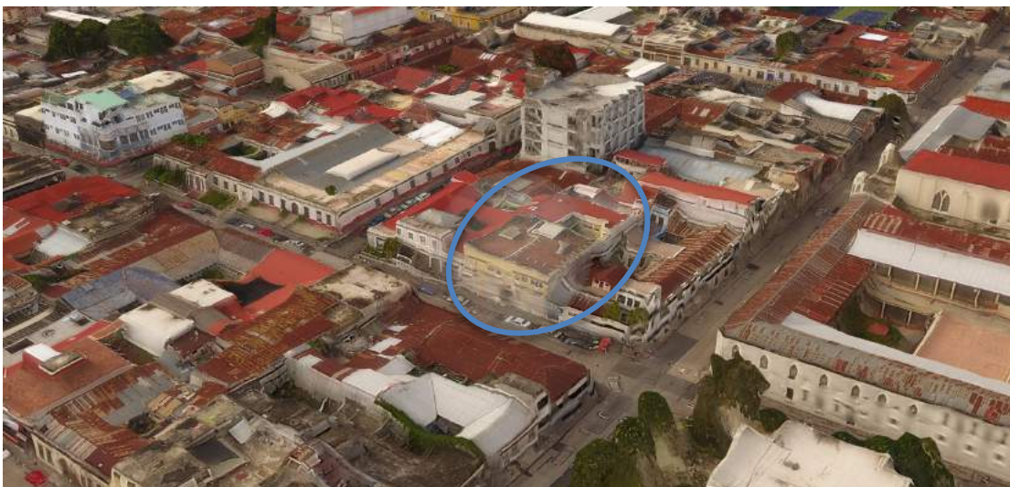
Figure P-11 Building 2: Drone 3D model - The Instituto de estudios comparado ciencias penales de Guatemala from the north west
