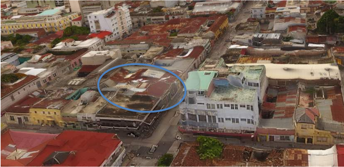
Figure L-4 Building 1: Drone 3D model - Colegio Mixto Santa Sofia from the south west
