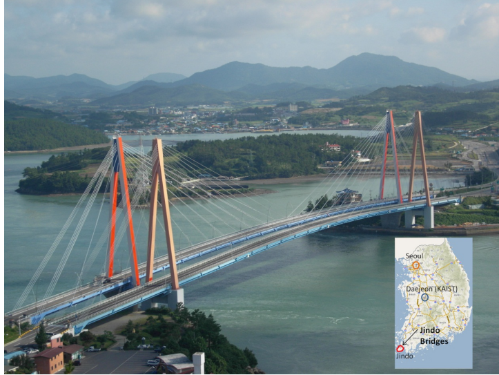
Figure 3.1: Twin Jindo Bridges connecting Jindo Island with the Korean Peninsula.
