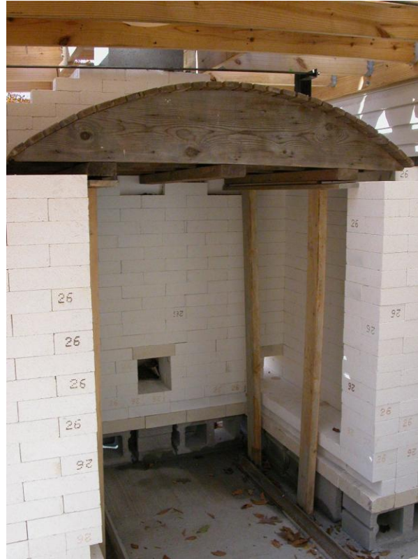
Figure 6.3. Wooden support system spanning the exterior walls.
