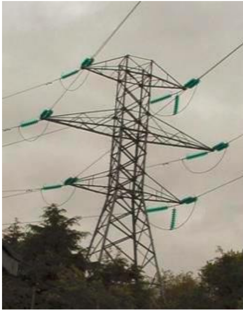
Fig. 2-3. Strain (angle) structure [19]
