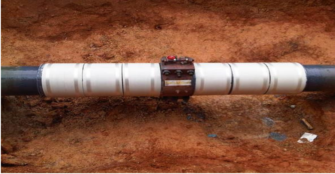
Figure 10. Crack repair using crack arrestors [163]
