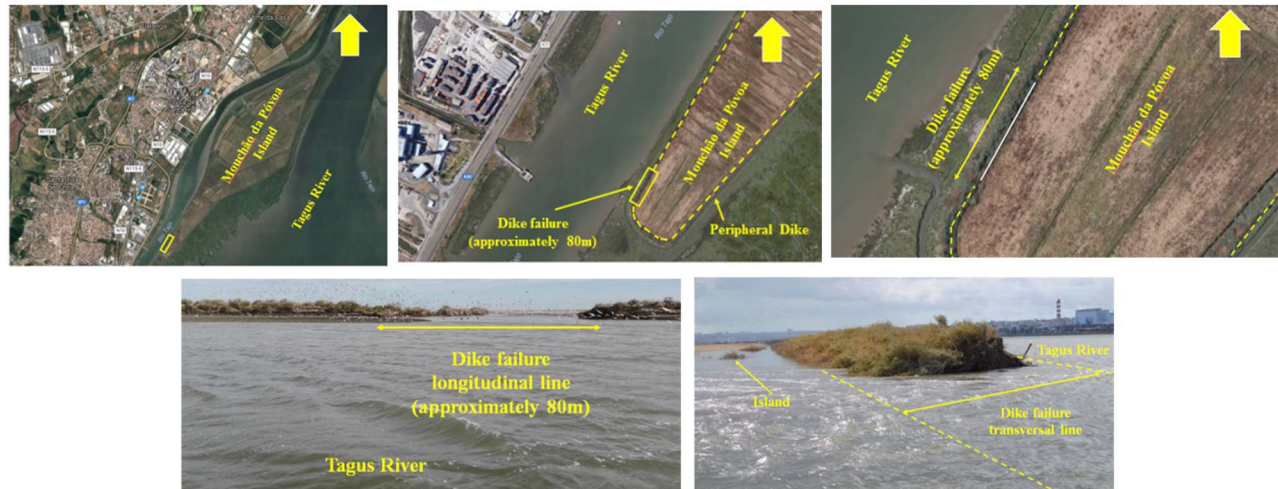
Figure 38. Location and view of the dike failure.
