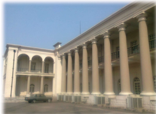
Figure 2: Long and deep verandahs as a shading device
