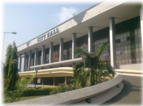
Figure 5: The deep roof overhang of the hall Source: Researcher's field survey, 2012
