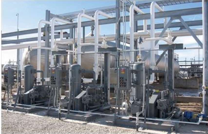
Figure 2-6 Multistage reciprocating compressors for liquid gas transfer (Source: Corken Company)
