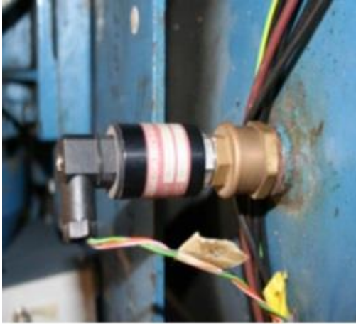
Figure 4-7 Static pressure sensor on air storage tank
