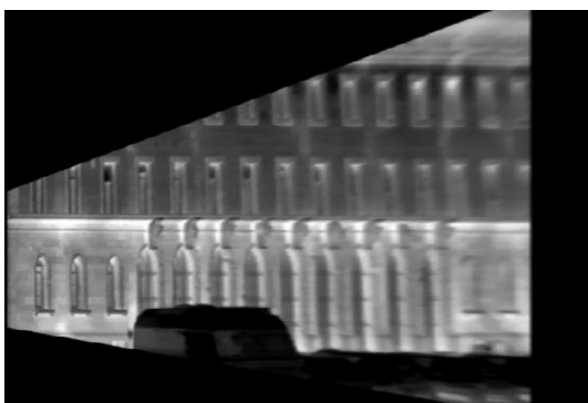
Figure 6. Partial texture of one façade extracted from one IR image
