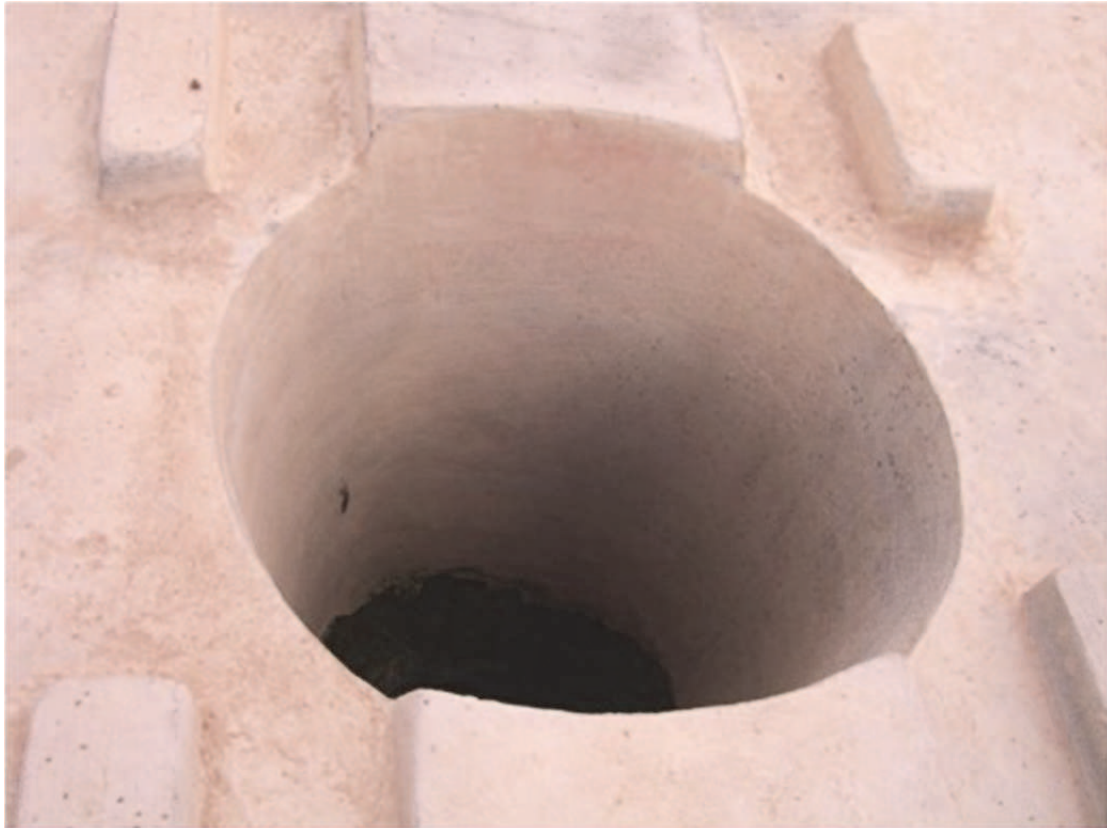
Figure 7 Shallow well apron design that accommodates traditional Somali water collection method of two large branches to be used effectively.
