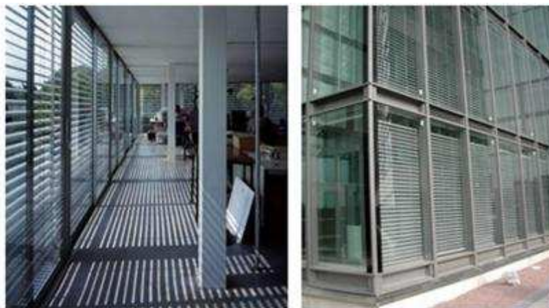
Figure 8-2: Examples of buildings with DSF system
