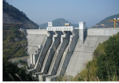
FIGURE 4: The downstream view of the concrete gravity dam.
