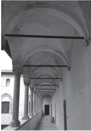
FIGURE 1: Tie-rods in the Castle of Torrechiara in Langhirano, Parma, Italy.
