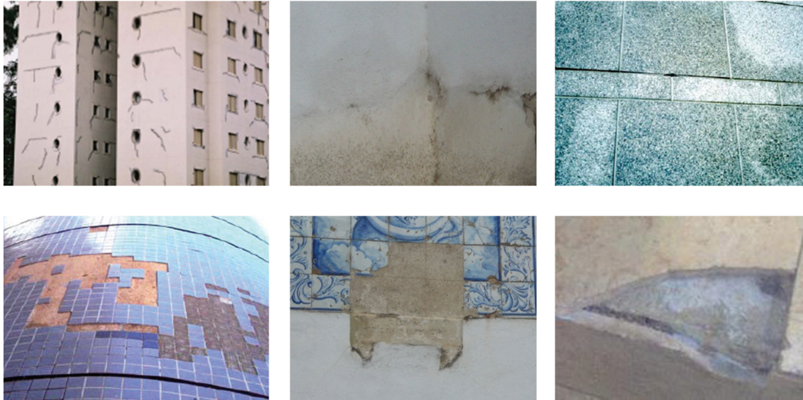
FIGURE 9: Different types of materials applied as façade coatings and some irregularities.
