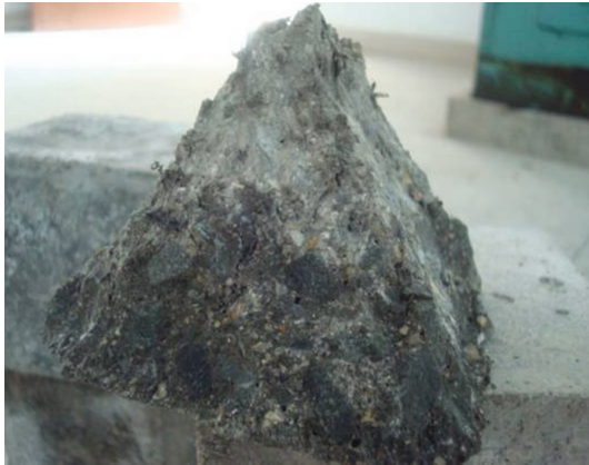
FIGURE 1: Damaged C120 concrete.
