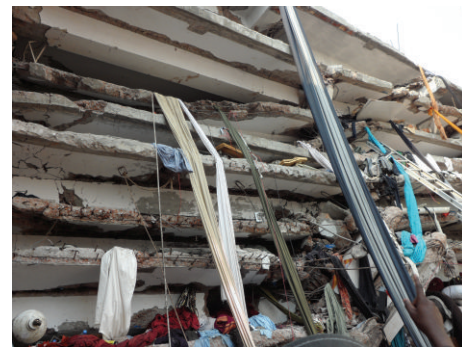
FIGURE 3: What happened after Rana Plaza collapsed.
