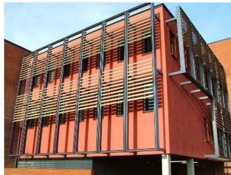
Figure 6 Hendon Magistrate Courts, fixed solar shading timber Louvers [15]
