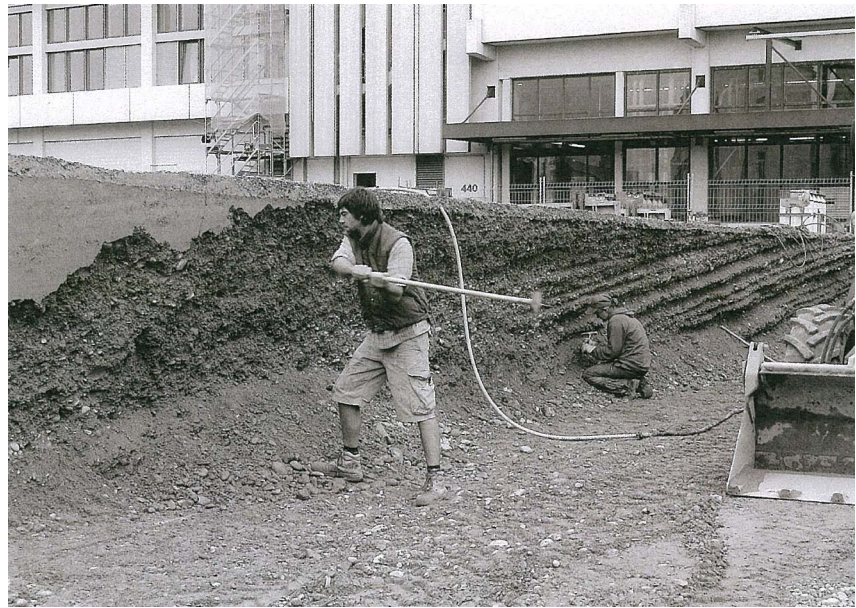
Figure 25. Vogt, Novartis embankment construction, Basel, 2006
