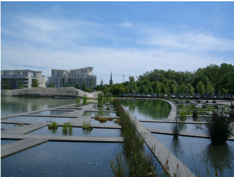
Figure 19. Constructed wetland in the Bordeaux Botanical Garden, 2005
