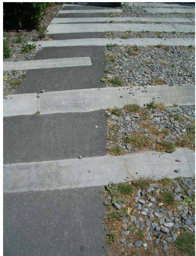
Figure 45. Entry ramp, Bordeaux Botanical Garden, 2005
