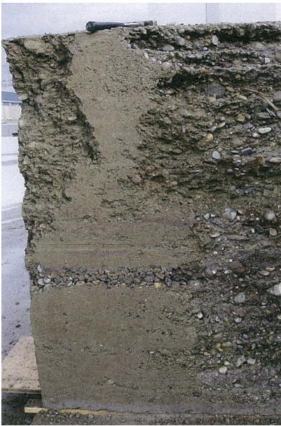
Figure 24. Vogt, Novartis embankment construction, Basel, 2006
