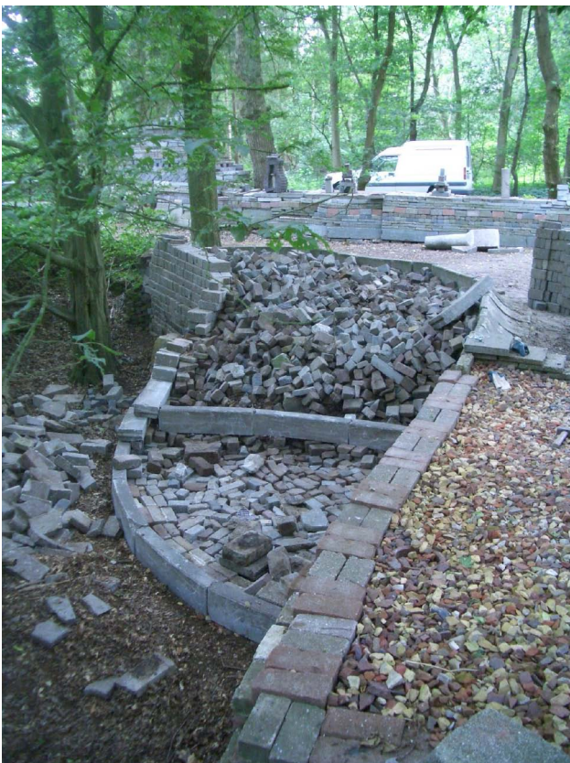
Figure 116. Step construction, Ecocathedral, 2007
