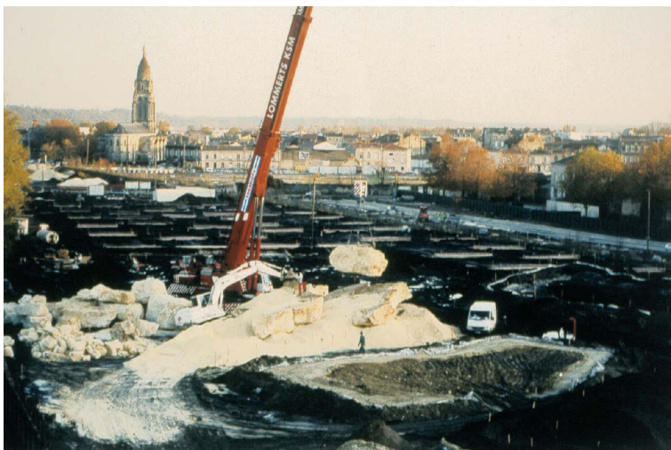
Figure 37. Construction underway at Bordeaux Botanical Garden, 2000
