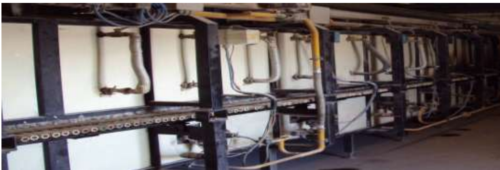
Figure 53 – Kiln 1 on the factory.
