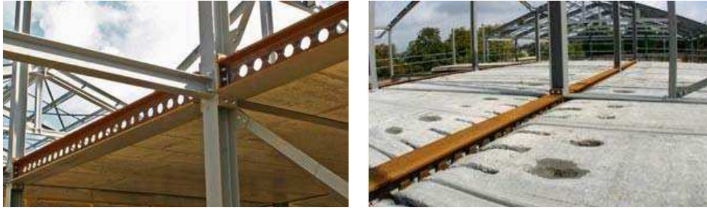
Fig. 2: USFB™ used with precast
