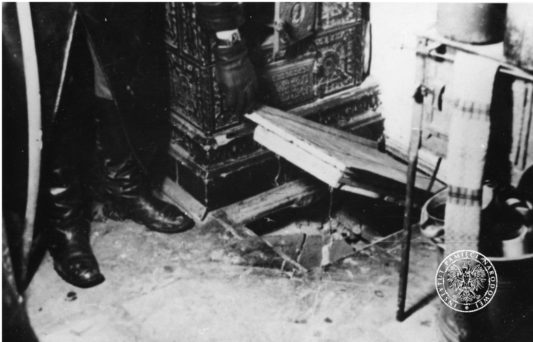
'Entrance to the cellar. Protective plate in front of the oven was nailed to a multi-layered wooden trap-door, thereby sealing off the entrance and rendering it invisible' (Katzmann, 2002, p. 68) – photograph from the collection of the Office for the Preservation and Dissemination of Archival Records of the Institute of National Remembrance – Commission for the Prosecution of Crimes against the Polish Nation (IPN, BU, GK_22408) (© Copyright by The Institute of National Remembrance – Commission for the Prosecution of Crimes against the Polish Nation)
