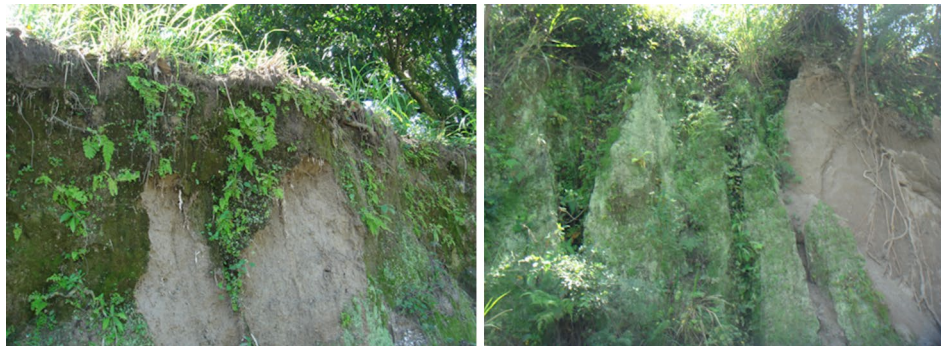
Fig. 6 TBJ slopes with the presence of biological soil crusts (BSCs) that protect on some level against mass wasting
