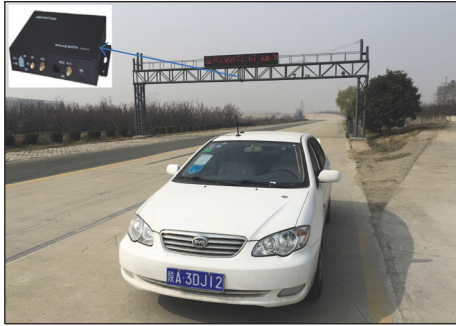
FIGURE 2: The DSRC RSU on the test-bed.
