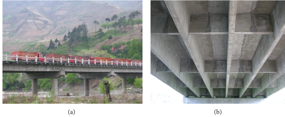
FIGURE 3: Overview of Nanping Bridge.
