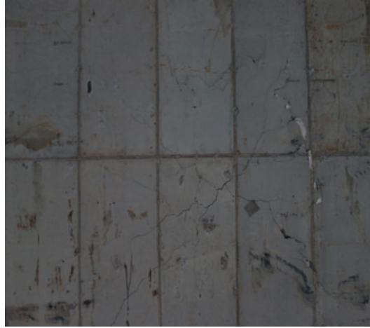
(g) Failure in FP-PT-xy specimen
