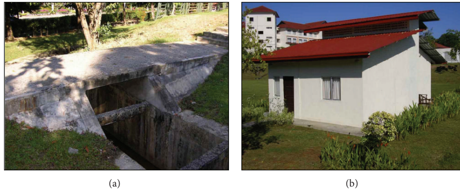
FIGURE 3: (a) Footbridge and (b) low cost house constructed using OPS concrete [16].
