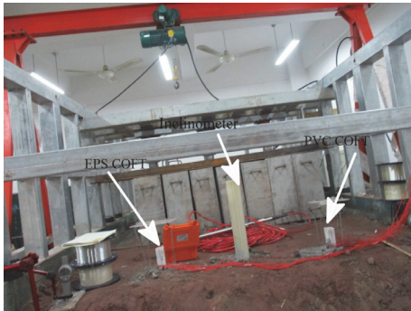
FIGURE 9: Photograph of the installation of COFTs and inclinometer.
