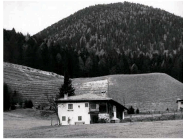
Fig. 3. 1981–1982: bottom view of the two basins almost completely replanted. It is possible to notice the progressive levels of growth achieved by hydrocyclone and the caretaker's house in the foreground (courtesy of Fondazione Stava, 1985).
