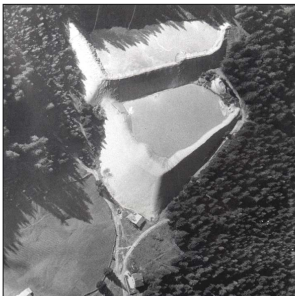
Fig. 5. Aerial view of the basins in October 1973, nearly two years after the construction of upper basin; in this one is in progress the raising of the embankment from the orographic left side (photo Impresa Rossi, Brescia).
