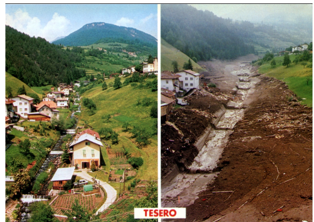
Fig. 13. Before and after the passage of the mudflow in the Tesero village at section 20 in Fig. 8 (postcard – Foto Trettel, P., edited by: Artesan, Tesero).
